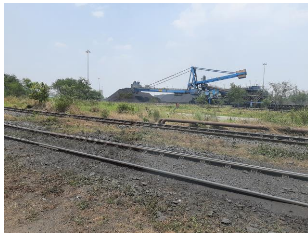
Coal Handling Plant
