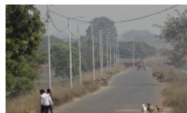
15 km long LED Street lighting covering 4 Gram Panchayats
