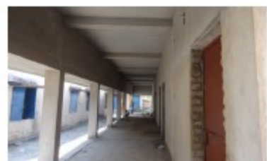
Construction of a school building nearing completion
