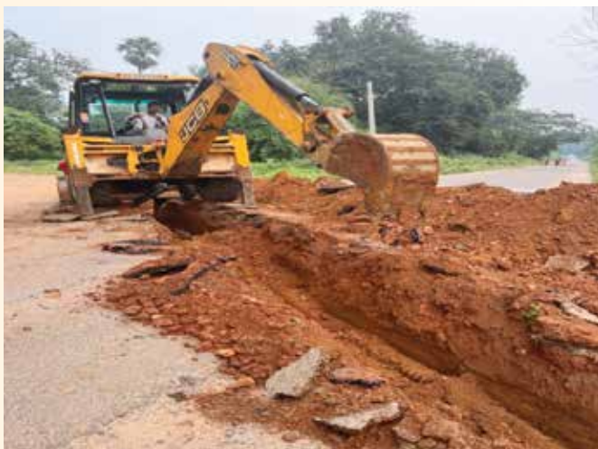
Laying of Drinking water pipeline to Periphery Villages of IB Thermal Power Station
