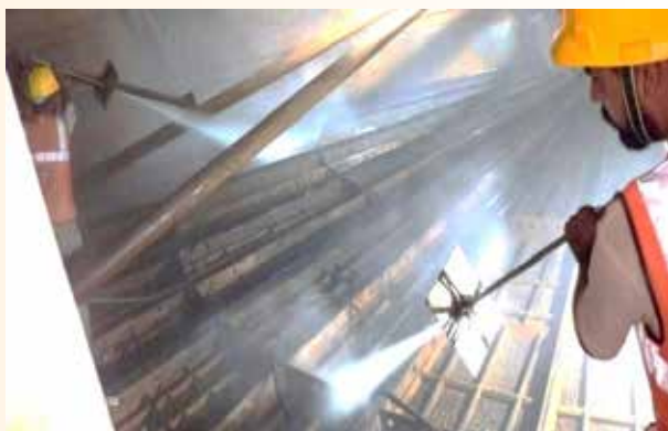
APH High pressure jet cleaning
