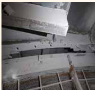
BEFORE PA hot end bypass seal was missing at some location
