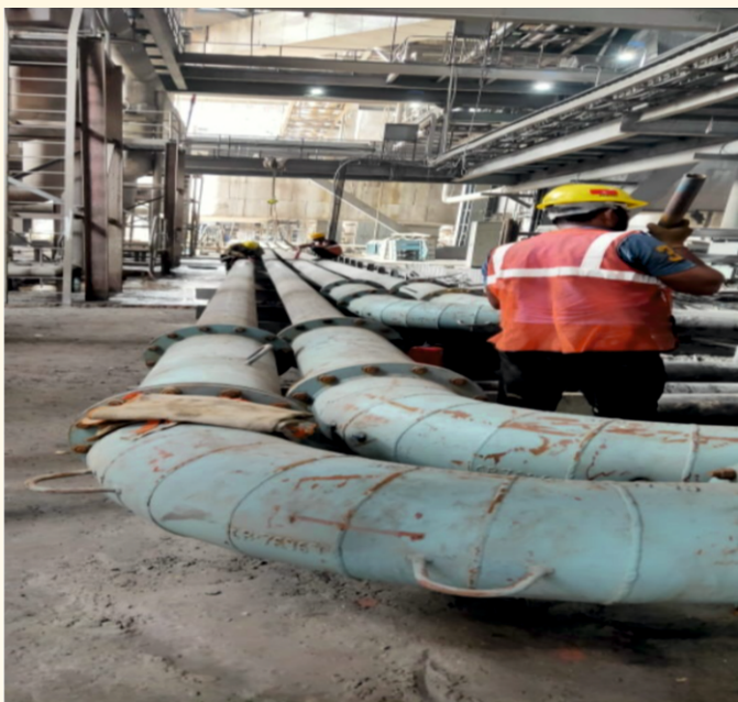
250 Nb size BA discharge line welding u/p
