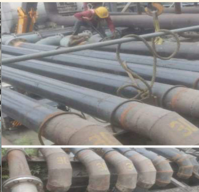
BA discharge line laying near slurry sump u/p
