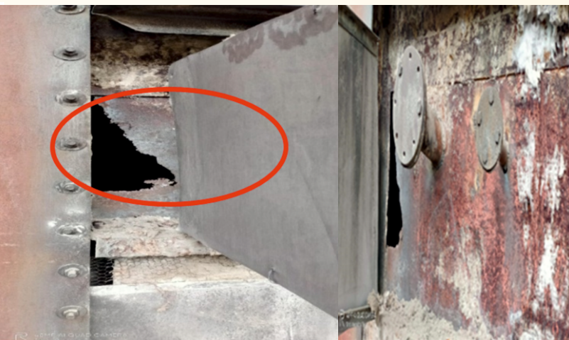
Damaged APH Duct
