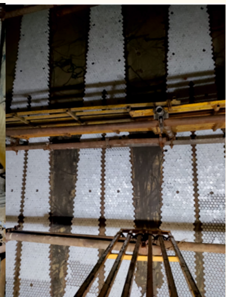
Ceramic coating in water box
