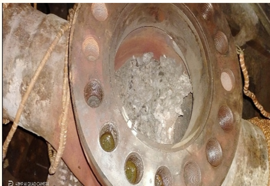
(AFTER) Valve body repaired and new design internals are installed
